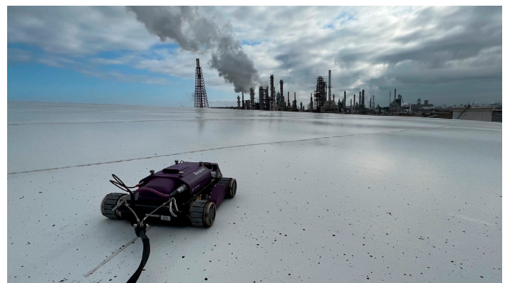
Figure 9: Scorpion 2 inspecting tank roof.
