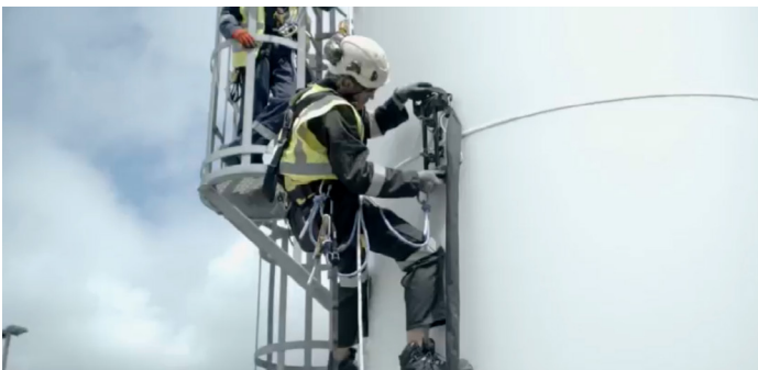
Figure 4: Rope access deployable solutions.
