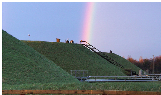
Semi-buried bulk fuel storage tanks
